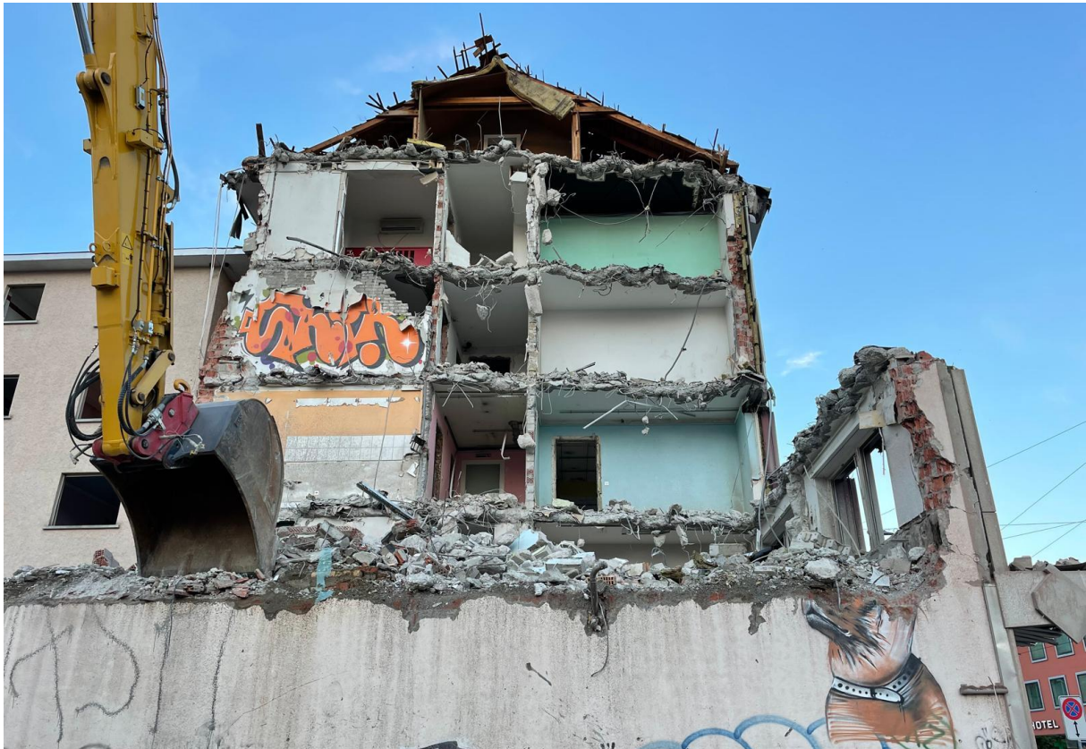
Fig. 5: Demolition of housing in Altstetten (Photo: J.Duyne, 2024)
