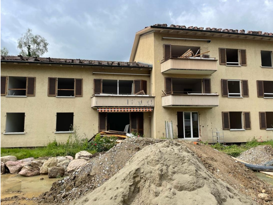
Fig A4.7 : Old low-density cooperative housing being demolished in Altstetten, 2022 (Photo: J.Duyne)
