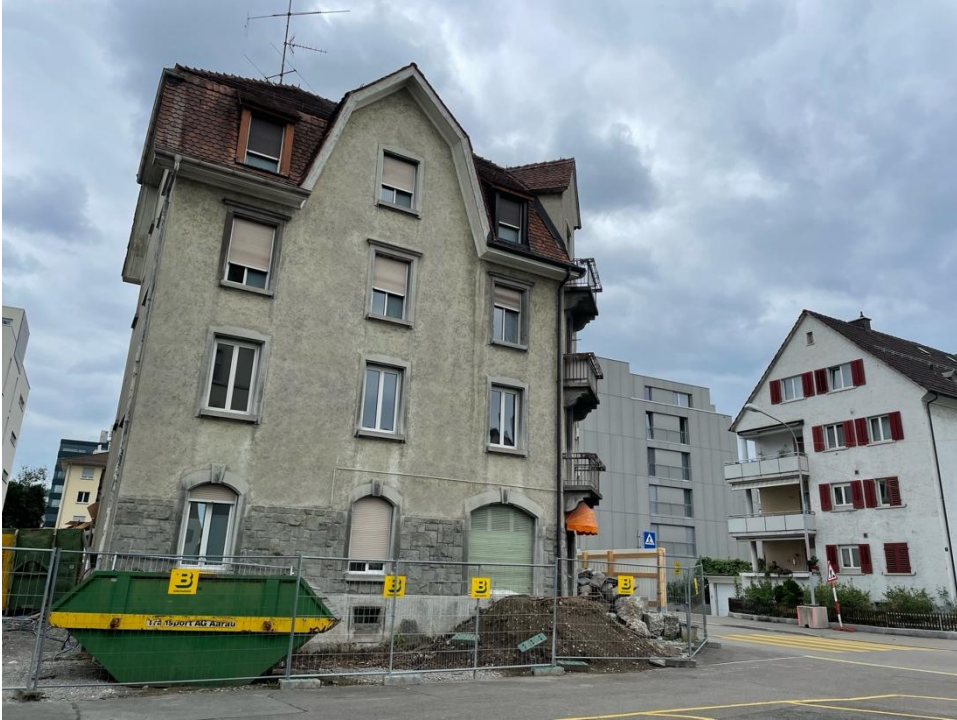
Fig. A4.5: Bachmattstrasse 39, Altstetten, 2023 (Photo J.Duyne, 2023)
