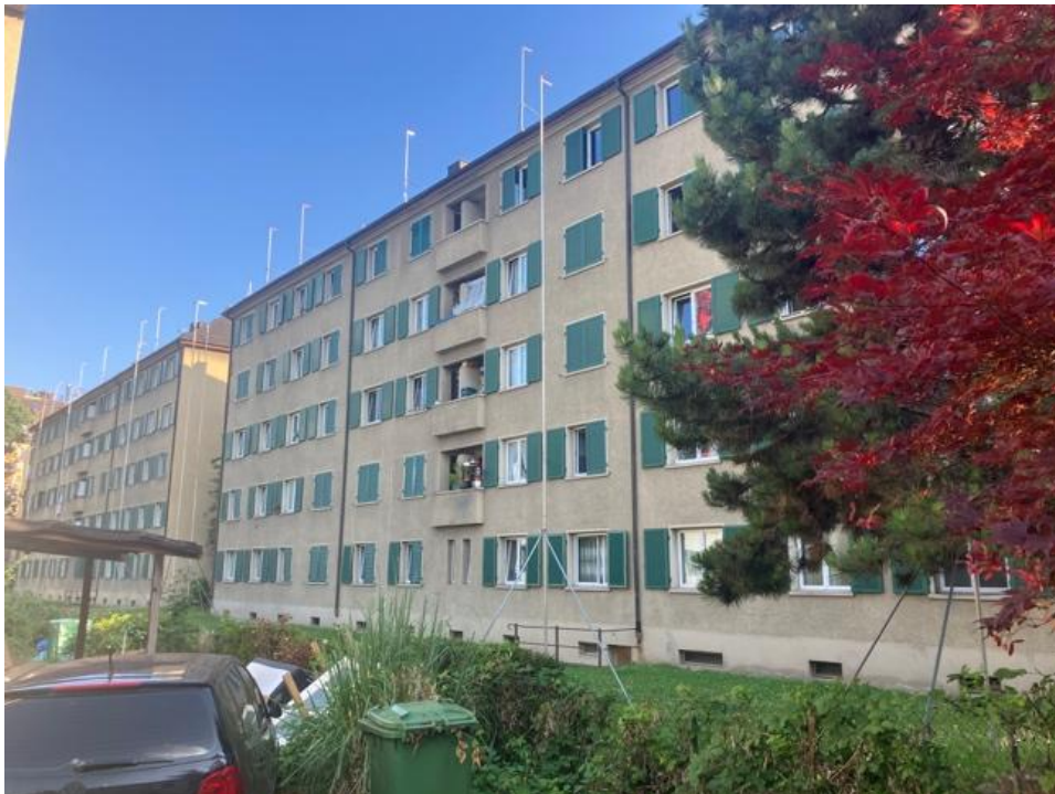
Fig. A4.2: Housing to be demolished for redevelopment in Altstetten (Photo: L. Gehrig, 2025)
