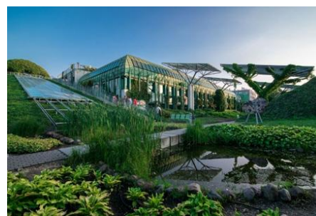
Figure 11: The garden on the roof of the University of Warsaw Library in Powiśle. Source: Warsaw Tourist Organisation (accessed on 13-01-2026: https://go2warsaw.pl/biblioteka-universytetu-warszawskiego/ ).
