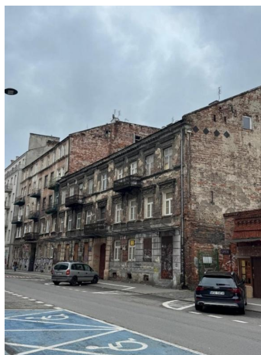
Figure 17: Historic buildings of Stara Praga – Brzeska Street. Source: T. Mikołajczyk (20-11-2025).
