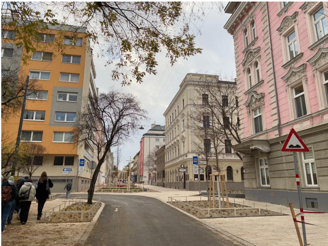
Figure 9: Supergrätzl with traffic circulation control and greening measures. Source: Judith M. Lehner
