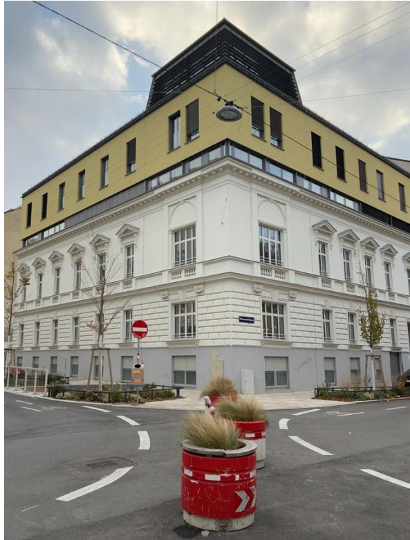
Figure 8: Densification through attic conversion (private building stock) and Superblock measures with traffic circulation control and modal filtering in Innerfavoriten. Source: Judith M. Lehner
