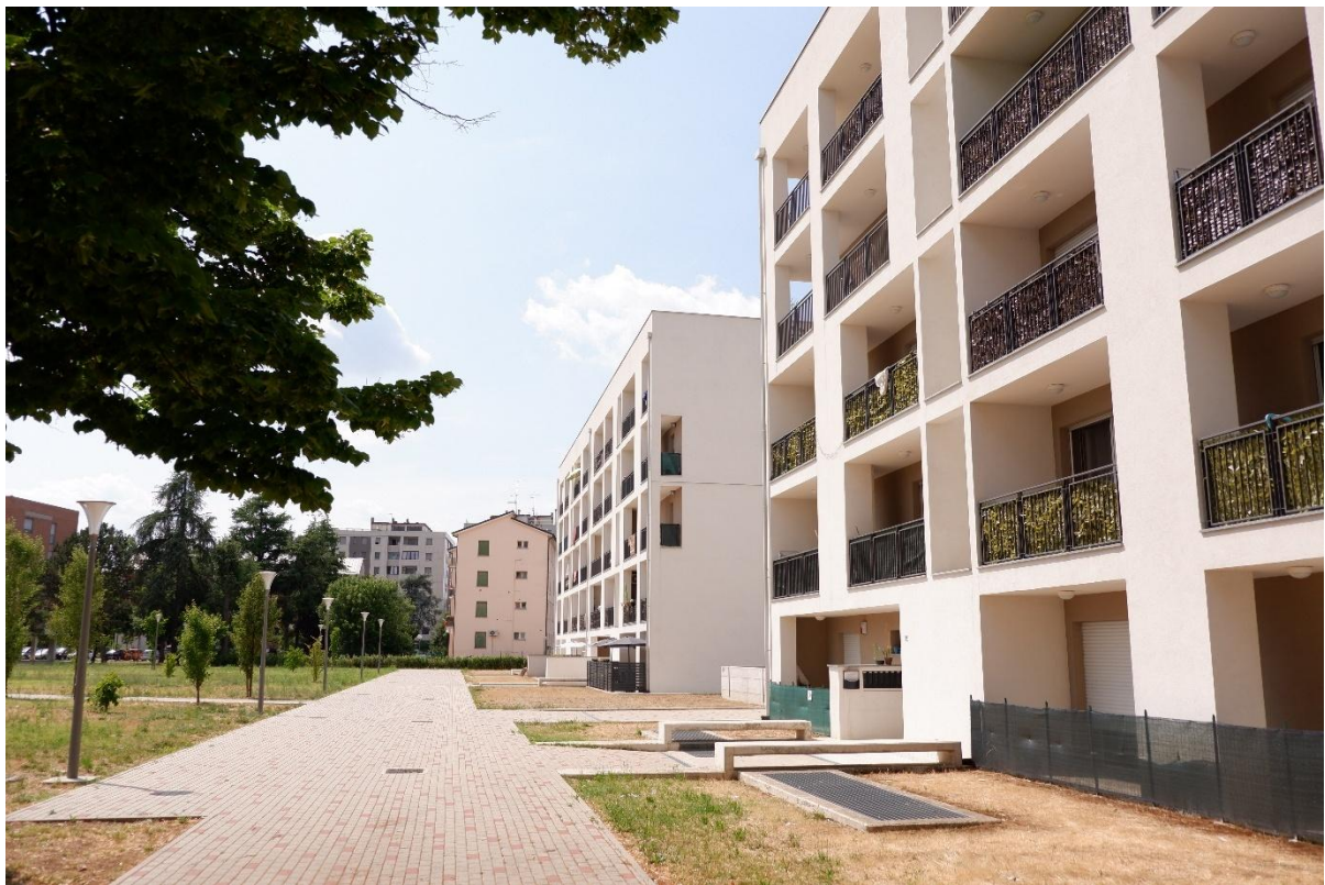
Fig. 8. Rebuilt public housing estate, Compagnoni neighbourhood, photo by authors
