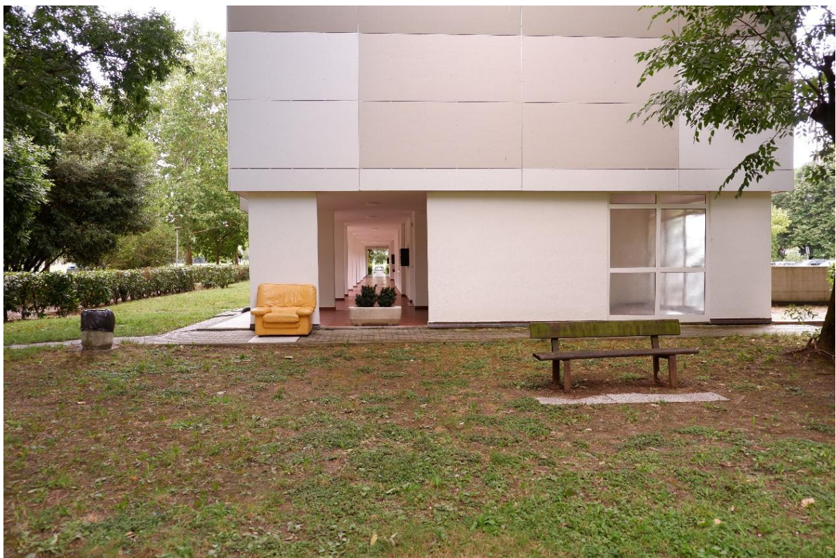
Fig. 14. Building after energy retrofit, Compagnoni, photo by authors
