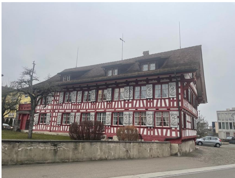
Figure 2: Vernacular house in Amriswil (© J. Duyne)
