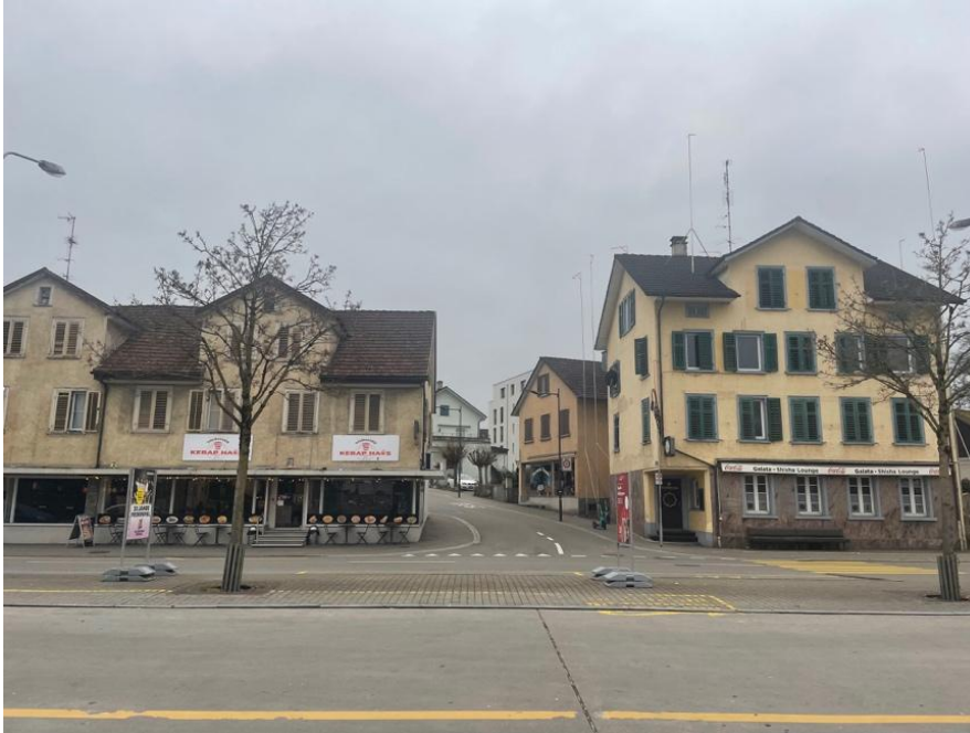
Figure 6: Buildings to be demolished at Bahnhofplatz (© J.Duyne)
