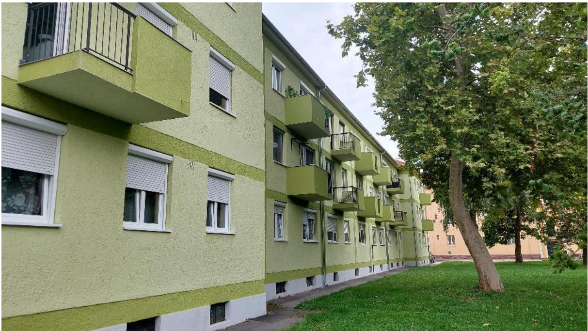
Picture 2. A building of the 1950s – painting without insulation (by Éva Gerőházi)
